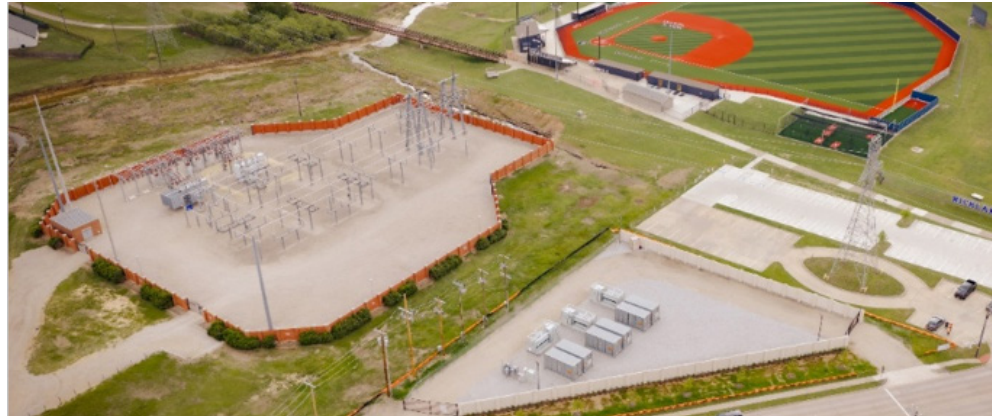
Meadow Park, a 12.9 MW / 25.8 MWh BESS microgrid demo site located in Dallas, Texas.
